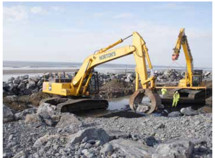
Borth Coastal Defence Construction
